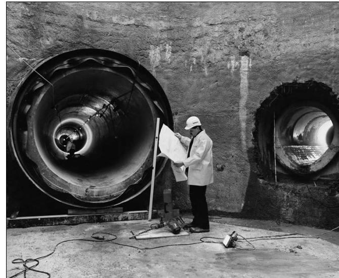
Figure 3.9 Construction of the sewer network.
