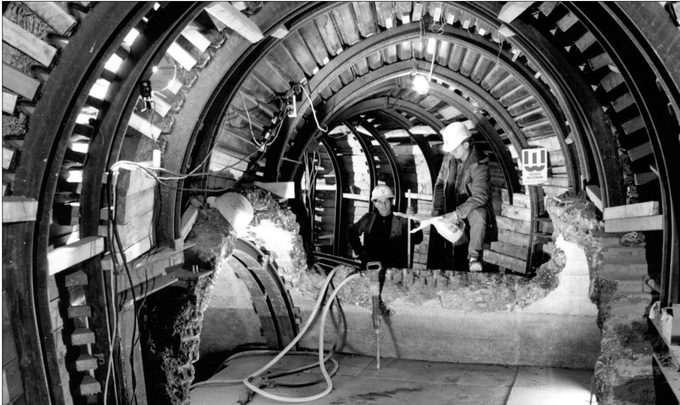
Figure 3.5 Sewer inspection and rehabilitation.
