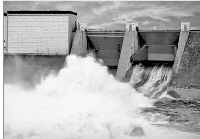
Figure 12.6 An Environmental Impact Assessment of a hydro-power plant. This EIA will consider the effects not only on the immediate surrounding but also on the river up- and downstream. The impacts considered will include ecological ones, e.g. biodiversity in the river stream; social ones, the consequences for those living along the river; and resource use impacts, e.g. the replacement of electricity produced from fossils with renewable energy. Photo: Vattenfall/Hans Blomberg.
