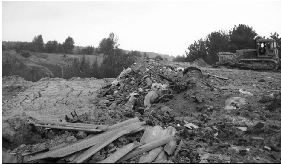
Figure 4.1 The landfill of the factory, which at the inspection received the mark “non-conformance” since it was not managed according to existing legal specifications.
