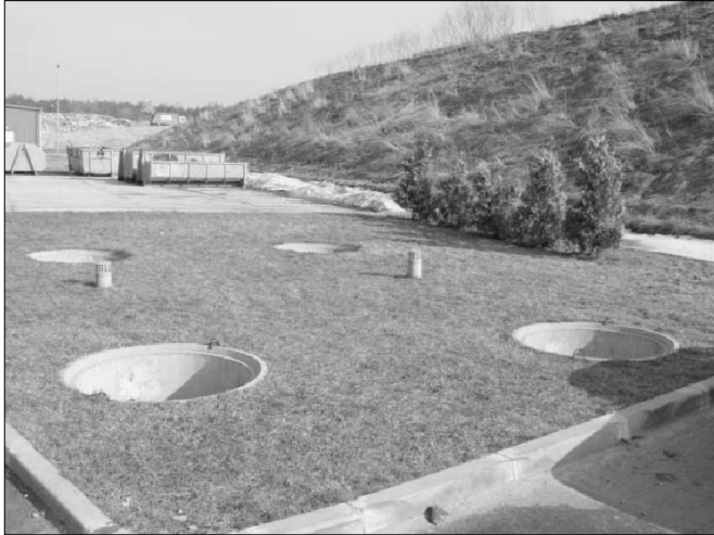
Figure 3.3 Tanks for leachate from landfill, composting plate for greek waste, and slope of old landfill.
