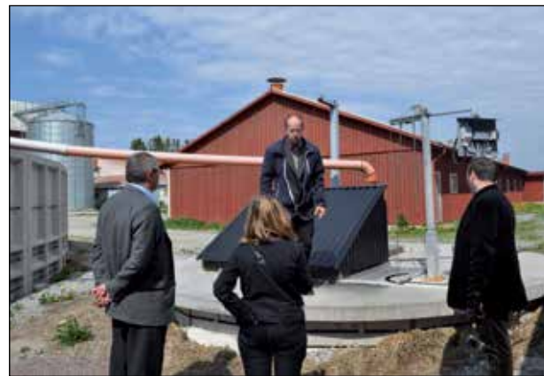
Figure 16.4. Biogas-production on the farm. This pig farm in mid Sweden, with an average occupancy of 3,000 pigs, use all manure for biogas production. The gas is used in a combined heat and power equipment, which provides all electricity and heat needed for the farm and a surplus sold to the electricity grid. To the right the anaerobic digester, also called fermentation tank. Photo: Lars Rydén.
