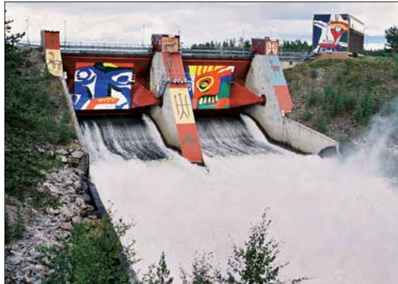
Figure 4.6. Akkats Hydro power plant by Lule Älv river outside the small city Jokkmokk in Northern Sweden. The mural paintings entitled Uvssat davás in the Sami language (Doors to the West) are made by Bengt Lindström och Lars Pirak. Photo: Hans Blomberg/Vattenfall.
