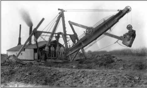
Figure 6.6. Dredge boat. To dig dredge ditches to drain farm land for drainage district. A slip scraper was used to dig hole in middle of field till there was enough water to float this boat. It was prefabricated and had a steam shovel in front to dig it's way toward the river. Taken into the field by wagons and put together on site. Building on back is crew quarters. Photo from Moultrie county in Illinois around 1900. Source: Illinois Digital Archives, made available by the Arthur Public Library.
