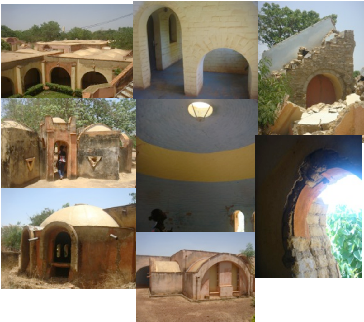
Figure 11 PID – Beautiful architecture but rapid and severe degradation
