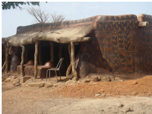
Figure 3 Kasena house in southern Burkina Faso made with wet loam stacking
