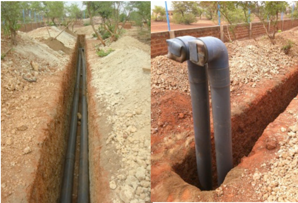
Figure 17 Earth cooling, air enters the pipes and cools down before it enters the house
