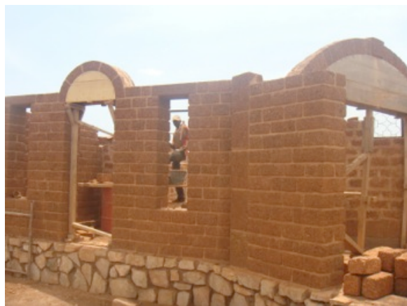
Figure 4 - House made of Pierre Taillé under construction in Ouagadougou
