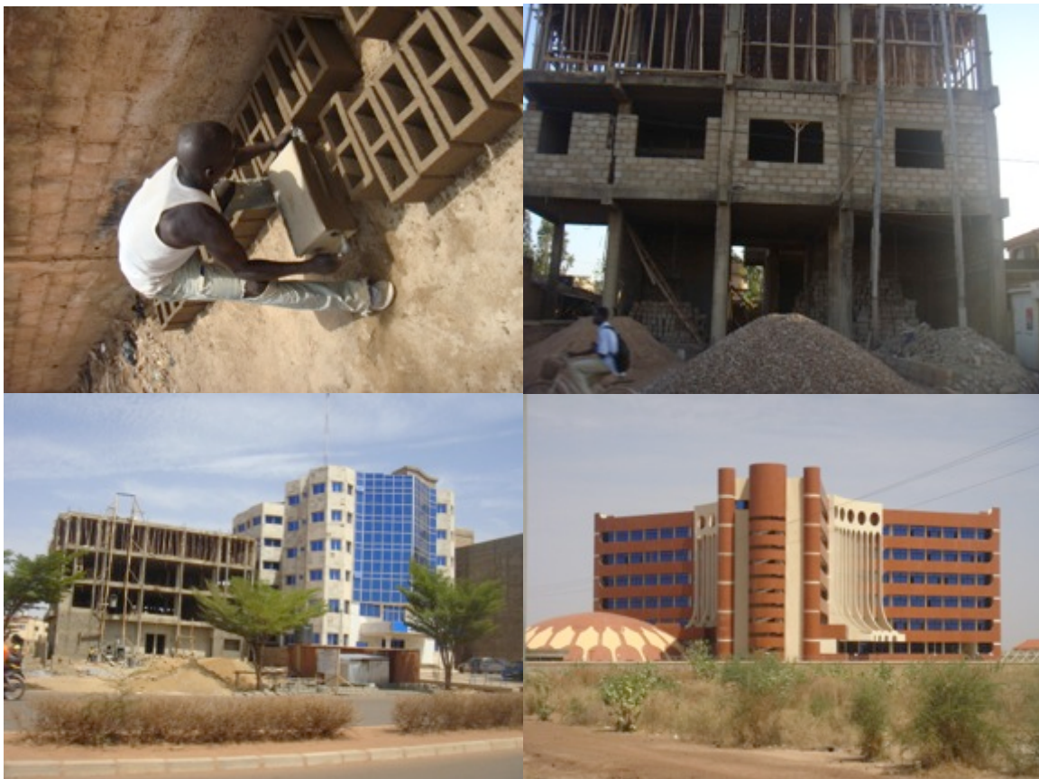
Figure 8 – Modern building with cement bricks and a load bearing concrete structure. Nice facades but no attention is paid to the thermal envelop. One air-conditioning system is instead put in every room.
